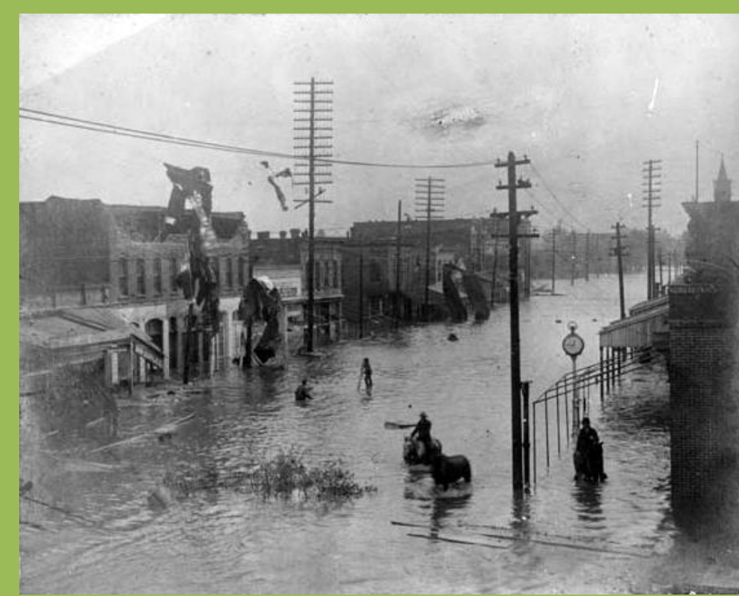
Brunswick, 1911, Storm Surge
